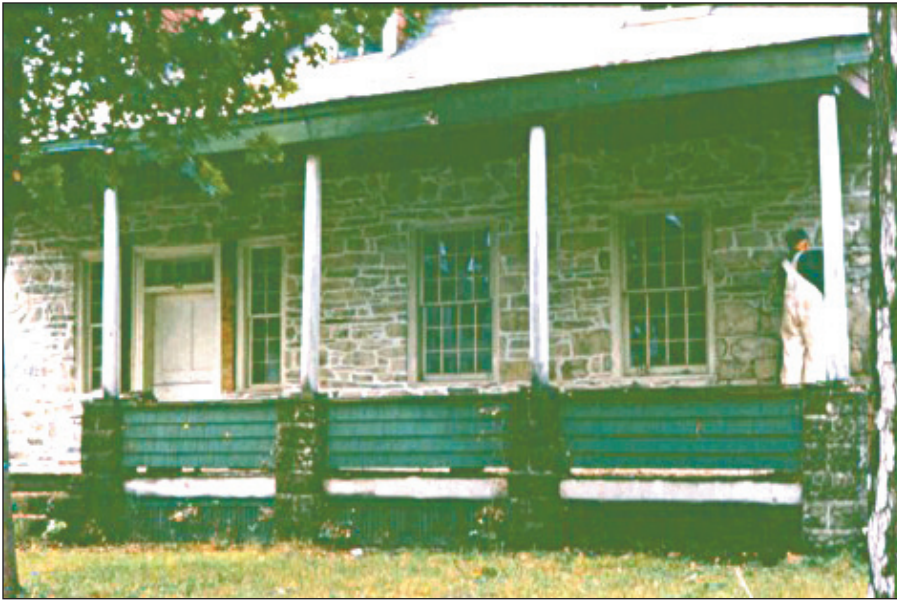
Restoration work began in the early 1960s.
