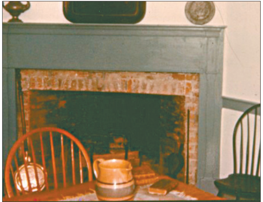
New brick works and a damper make the fireplace workable.
